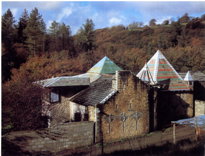
1--THE HOUSE FROM THE EAST. The walls are faced in granite rubble with granite quoins cut from curb stones. The kitchen dining bay shown in Figure 4 is on the left
