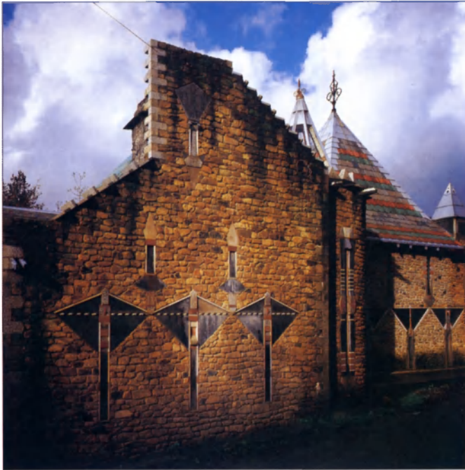
Barley Splatt (east facade), near Bodmin, Cornwall, begun 1973
